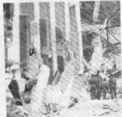
Highland Towers: Pronouncements on strict regulations are always an after-thought.
