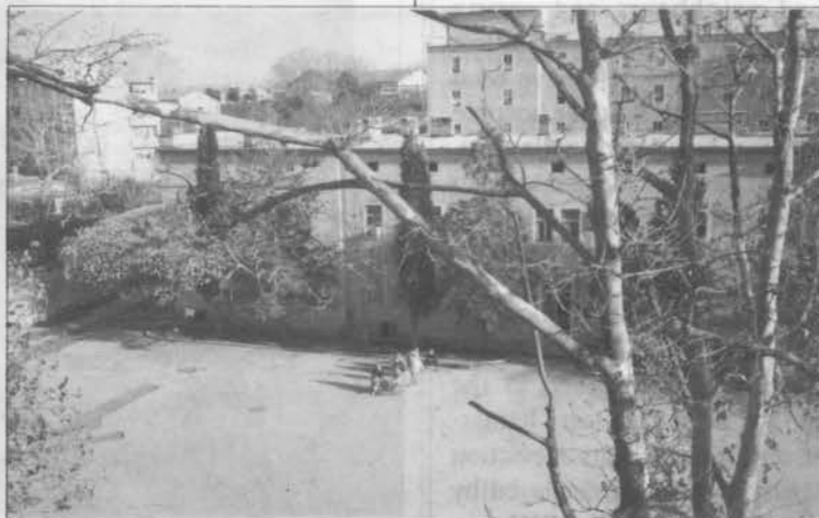
Invalids Centre Kamenjak, Pula. Picture of the courtyard between the 1st and 2nd (Invalids) Building.
