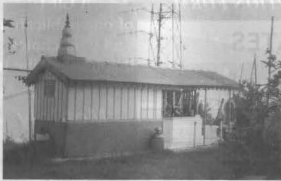
Before the destruction :The temple with its original shrine below the plaque
