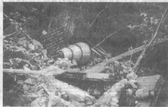
The remains after the demolition
